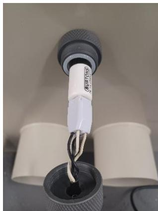
Loosen off the glad on the cable so the cable can move freely. This is important to stop the lamp from spinning around when you tighten the cap.
